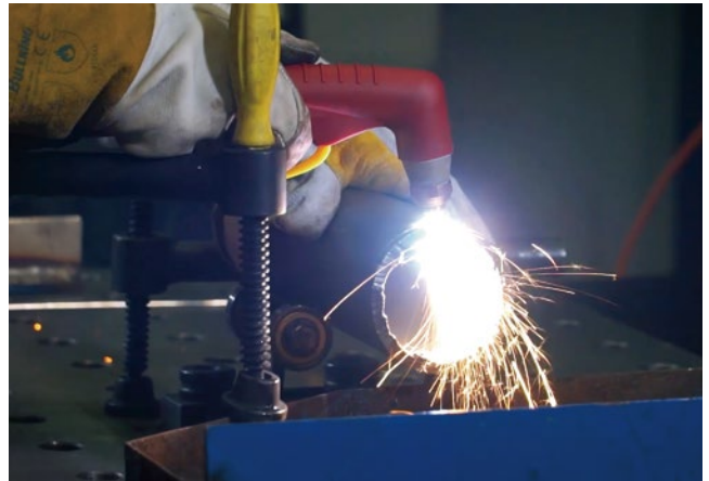
*90mm diameter, 9mm thickness pipe cutting by PROCUT-45MAX
